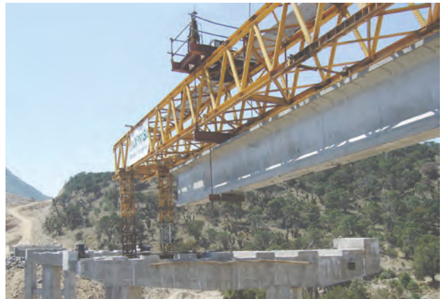
Tezontepec Bridge, Morelia-Maravatío Highway
