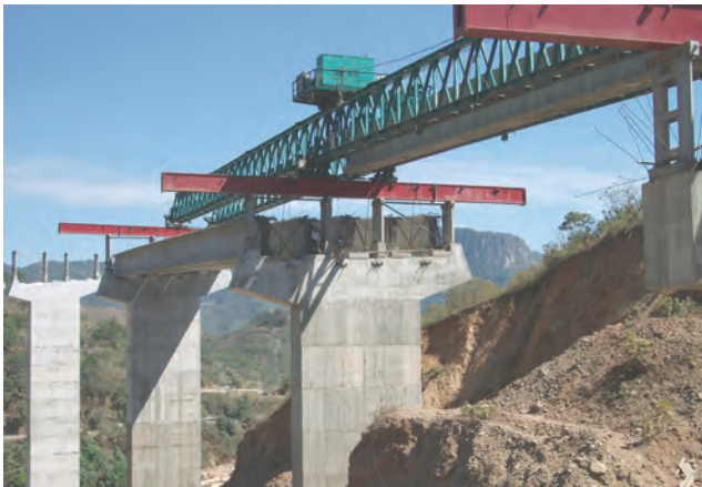
Nacaral Bridge, Durango-Mazatlán Hwy
