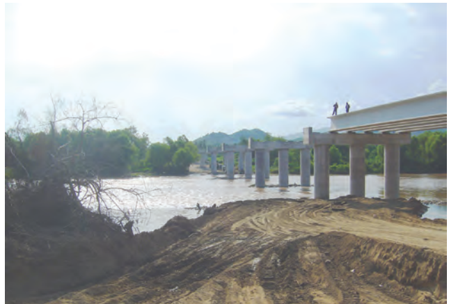
"Tecpan de Galeana" Bridge ,Quintana Roo
