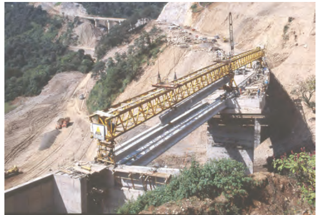
Maltrata Bridge Esperanza -Córdoba Highway
